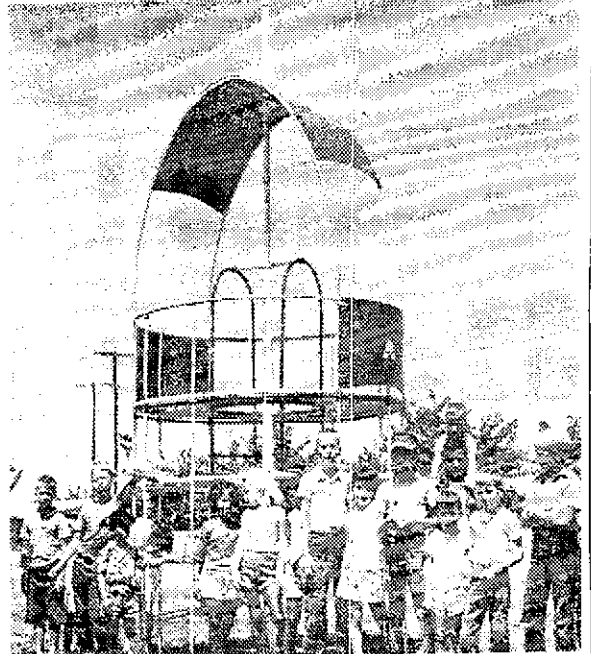
ENJOY SLIDE TOWER—A Castle Slide Tower has also been installed at Palm Grove park. Eager youngsters climbed aboard while a worker was still laying a cement base under the Tower.
