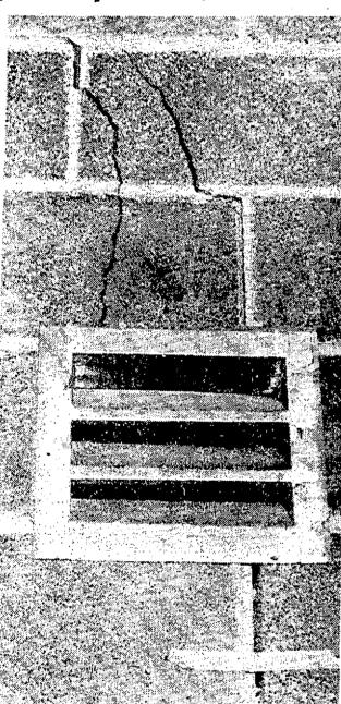
HUGE CRACKS through the cinder blocks around a ventilator in the east wall of the bull barn show the damage done by settling foundations. Concrete has been pumped under the building in an effort to halt the damage.
